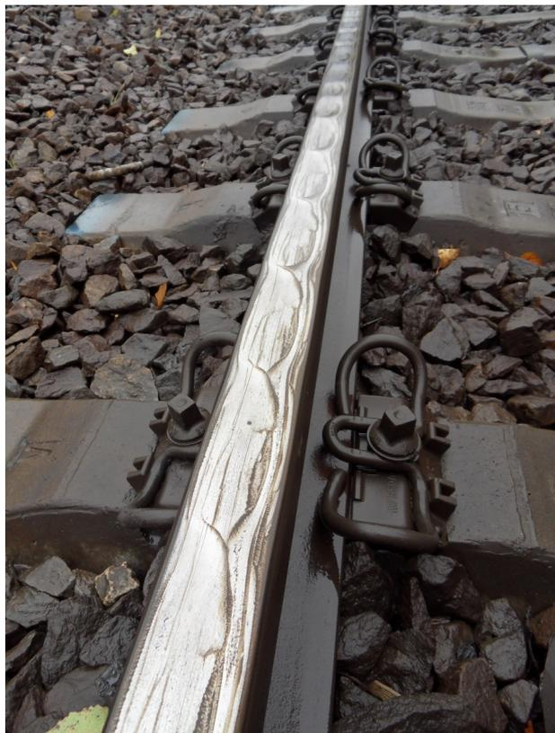
FIGURE 2. Highlighted long-pitch corrugation by contaminant in Havlíčkův Brod
