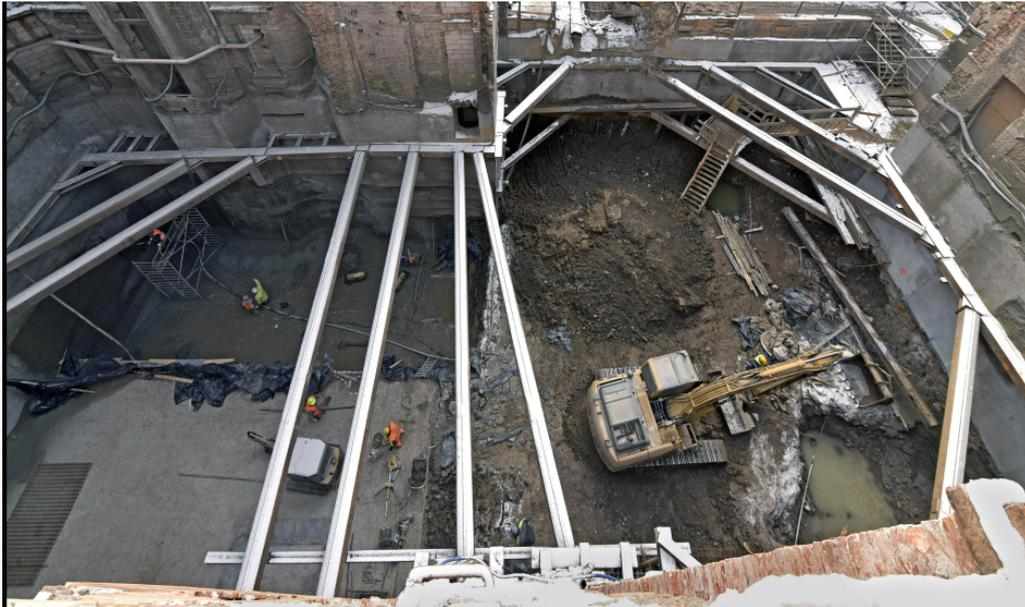
FIGURE 2. Construction pit – blinding concrete in process.
