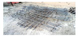
FIGURE 3. Y10 Beam Reinforcement.
